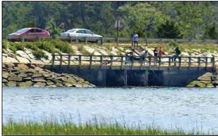
Figure 11. Existing Chequessett Neck Road Dike (Source: NPS 2011)
