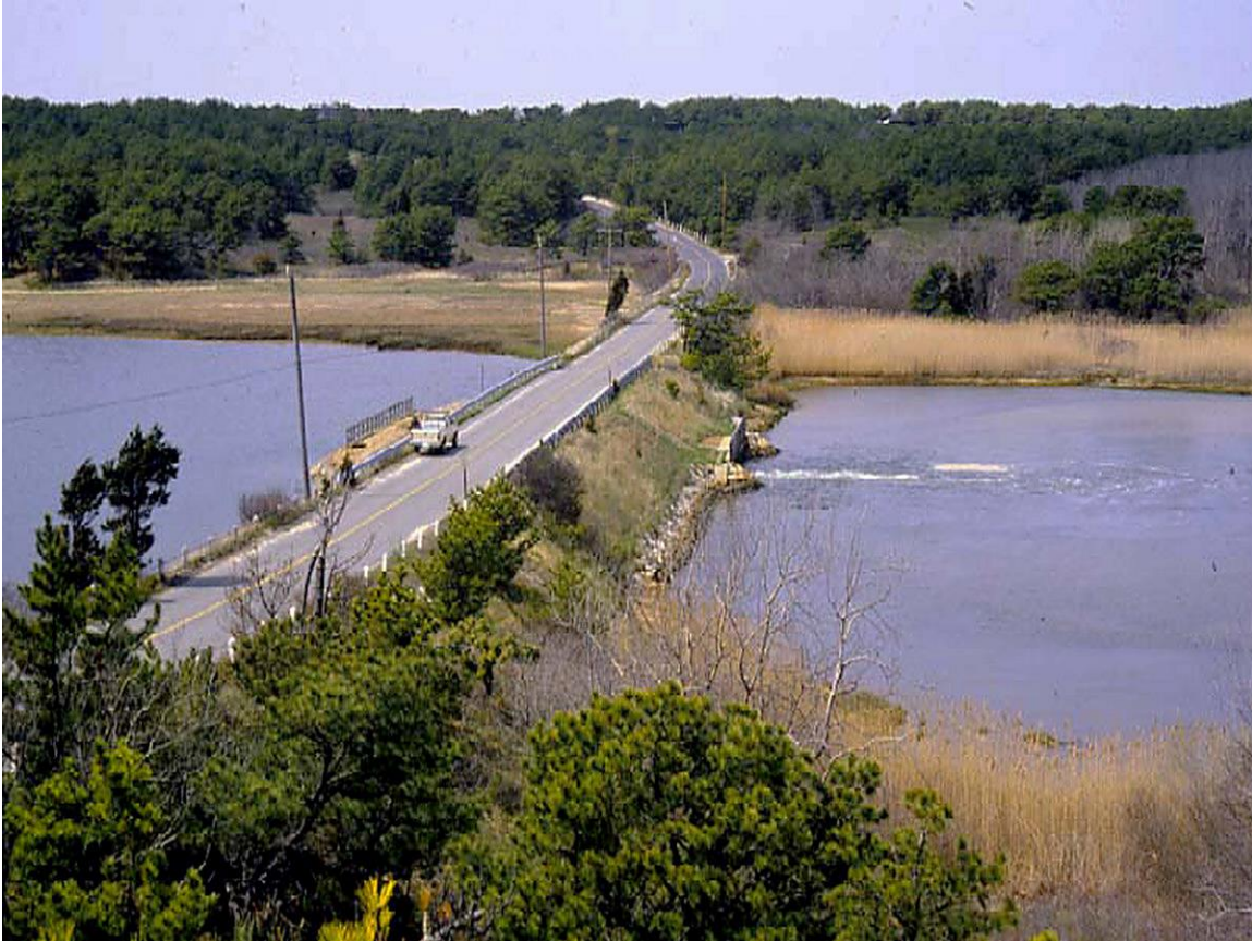
Figure 3. Chequessett Neck Road Dike today
