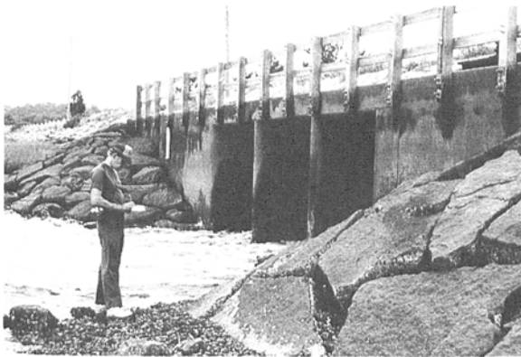
Figure 2. Dike and tide gates near the mouth of Herring River. Tidal range downstream of the dike (left) is 2.3 m and 0.5 m upstream (right). Note the three openings through the dike, fitted with a sluice gate and two flapper-type tide gates.
